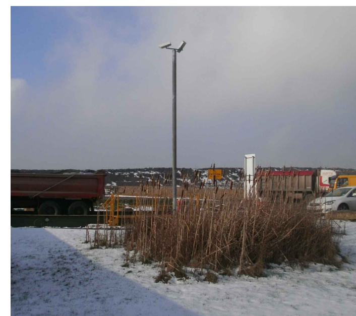
CCTV tower to the north east of the weighbridge
